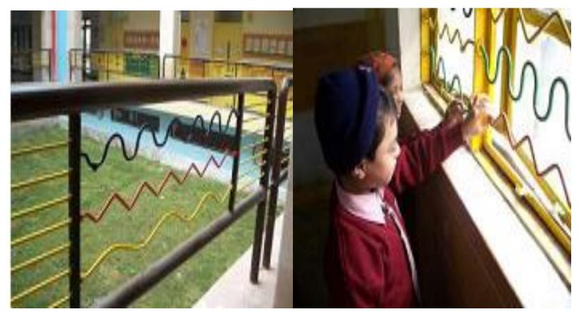
These metal window security grills or raining can be made at the time of new construction. The shapes have been worked out to prepare the gross and fine motor movement of the shoulder, elbow and wrist to prepare for writing various alphabets. Modification in existing grill needs to be done only upto the child accessible heights.
